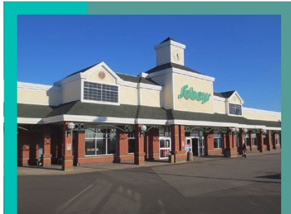
WOODLANDS CENTRE 300 THICKWOOD BLVD FORT MCMURRAY, AB
