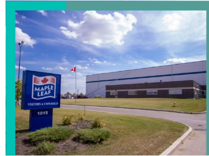
MAPLE LEAF BUILDING 53021 RANGE ROAD 263A SASKATOON, SK
