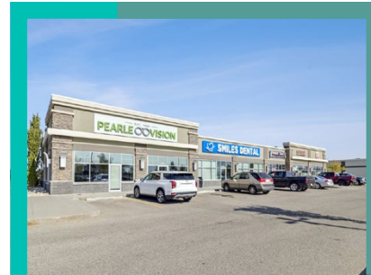
CENTURY CROSSING III 141 CENTURY CROSSING SPRUCE GROVE, AB
