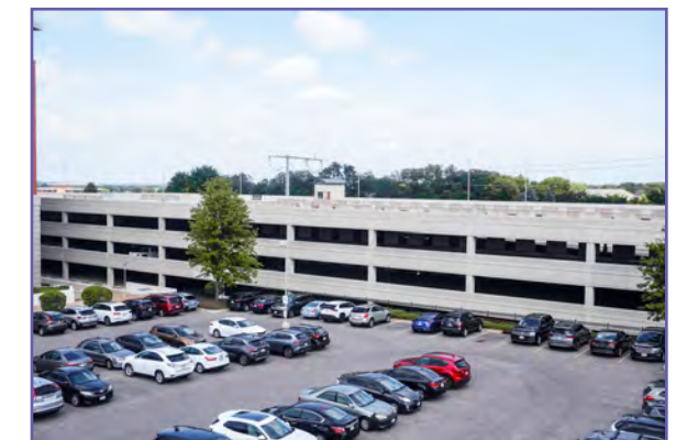
Covered Parking Ramp
