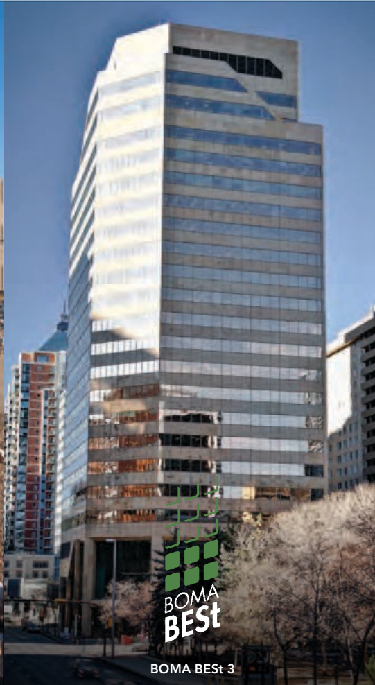
TRIMAC HOUSE / Calgary, AB
